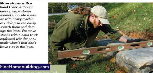
Keep water moving downhill. After we remove the sod and dig into the slope to accommodate the proper rise of each step, we lay down quarry dust to create a base for the stone. We build up the back of each step with dust to pitch it at least 1/4 in. per ft. If water ran back into the hill, it would freeze in the winter and cause the steps
