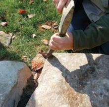
for a clean fit. With the first stone set, we choose a neighboring stone with an identical rise. With the front edges of both stones aligned, we scribe a line parallel to the first stone onto the second stone. A few shots with a chisel and a rock hammer make quick work of trimming the stone. Don't get carried away, though. Fill the gap between stones with quarry dust.
