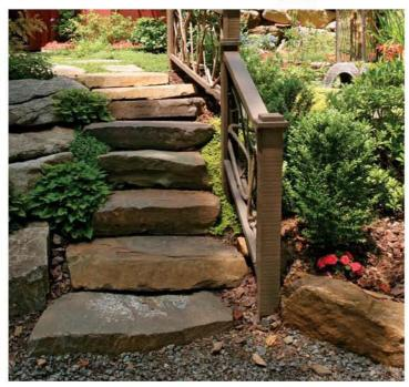
Skip the mortar, and use packed quarry dust for a walkway that will last a lifetime
