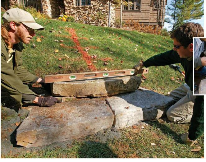
Leveling requires addition and subtraction. Because we're using rough stone, we sometimes need to add shims or to remove knots, or high spots, in the stones so that they rest soundly on each other. We use broken pieces of stone as shims to fill small gaps and knock down the knots with a chisel and a rock hammer.
