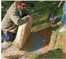
Surgery with sod and stone. As we move up to the top step, we place each stone where we want it for the appropriate run and scribe the back of it into the hill with a shovel. We remove the sod and dirt within the shovel line, then add a pad of quarry dust to level the step as needed. Once the steps are in, we replace bits of sod around the steps.
