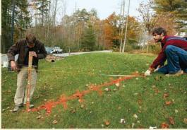
Indicate the step location with marking paint. When the paint dries, use a line level, a level, and a tape measure to determine the total rise and total run of the slope.
